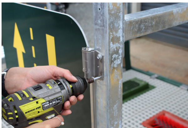
Ensure fasteners are secured tightly.
