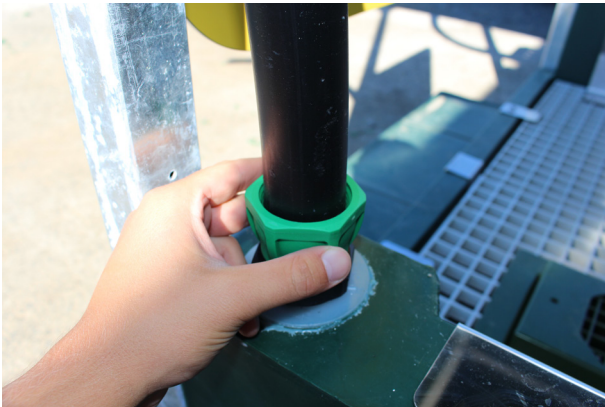
Check downpipe fittings and tighten accordingly.
