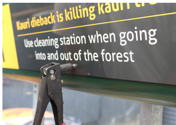
Ensure signboards are riveted on tightly.
