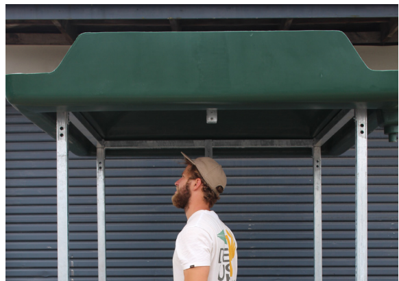
Look for any splits in the plastic of the roof.
