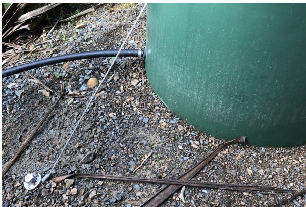
Check earth anchors are secure in the ground and the cables are taut on the tank.
