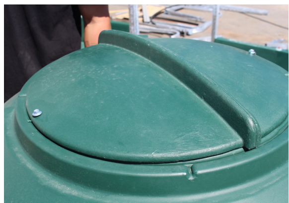
Check the tank lid is fastened down with two Tek screws.
