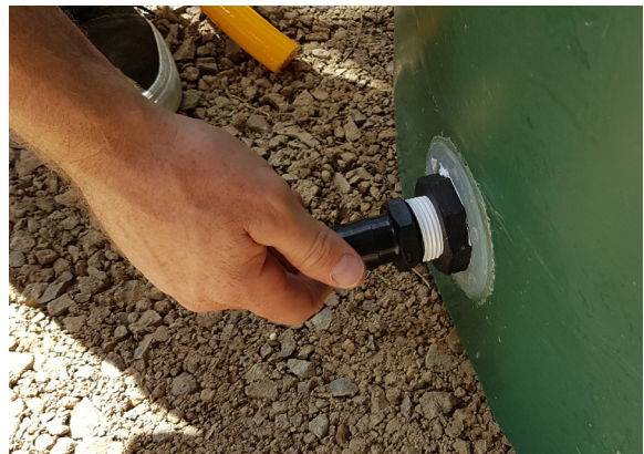
Check fittings attached to the tank. Tighten any if necessary.
