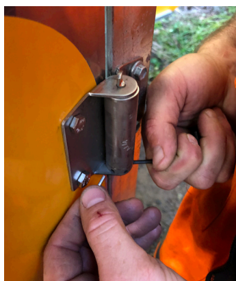
Remove the small stainless pin in the hinge then turn the hinge to the right again.
