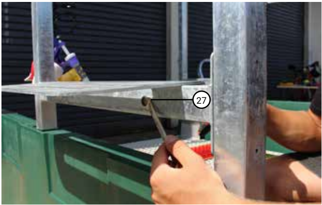
Thread a M8 Galv Nut onto the bolt and tighten using a 13mm spanner and a 13mm socket and wrench. Repeat on other handrail. Each seat should be next to the foot scraper/ footbrush on the mesh.
