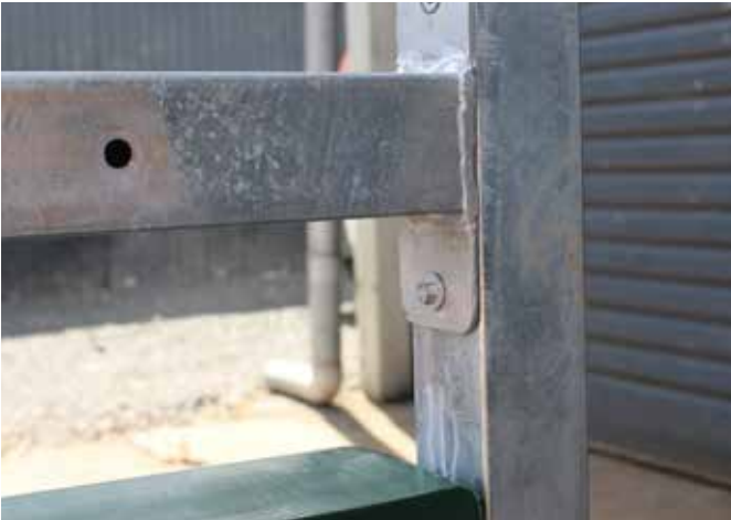
Using the power drill and TEK screw bit, fasten the handrail to the uprights.
