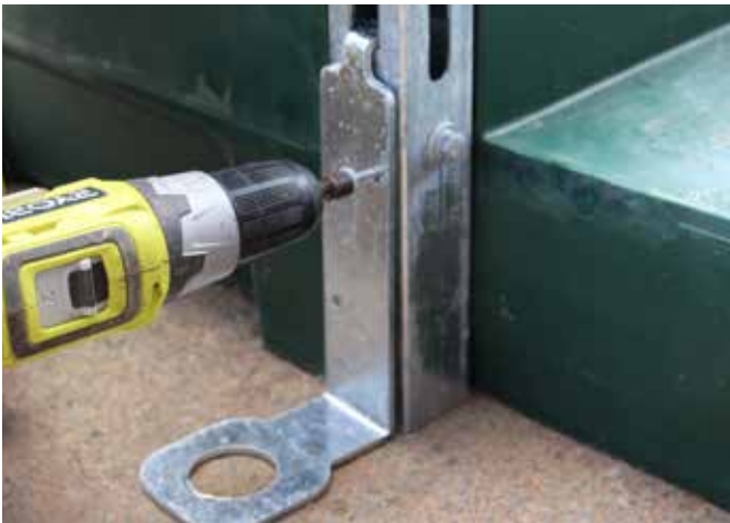
Use the power drill and 3/8" TEK screw drill bit to screw them into the upright. Repeat on the other hole of the bracket.
