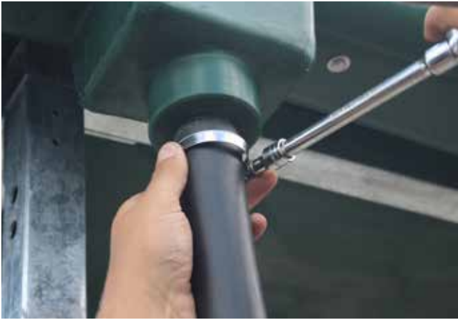
Tighten hose clamp with a 7mm socket. Ensure your pipe is cut square at each end at sits straight up and down, flush against the square drain filter box.
