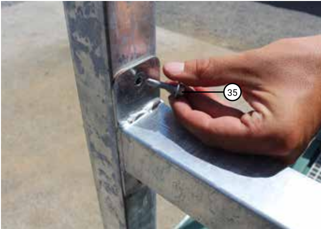
Line the ends of the handrail with the holes in the upright posts. Insert the TEK Screw tip into the holes.
