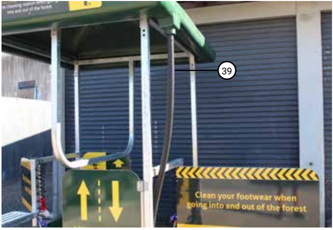
If your pipe is too long it will not attach correctly. Use 2 x large cable ties to secure the downpipe to the upright.
