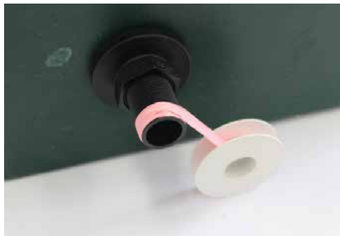
Thread tape the end of the male tank fitting thread.
