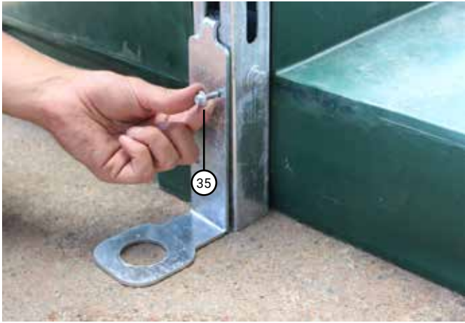
Insert the tip of a TEK screw into one of the holes on the earth anchor bracket.
