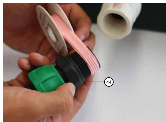
Thread tape the end of the 25mm male coupling.
