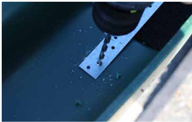
Using a 6mm drill bit, drill out the second hole in from each end of the strap, through the roof plastic too.
